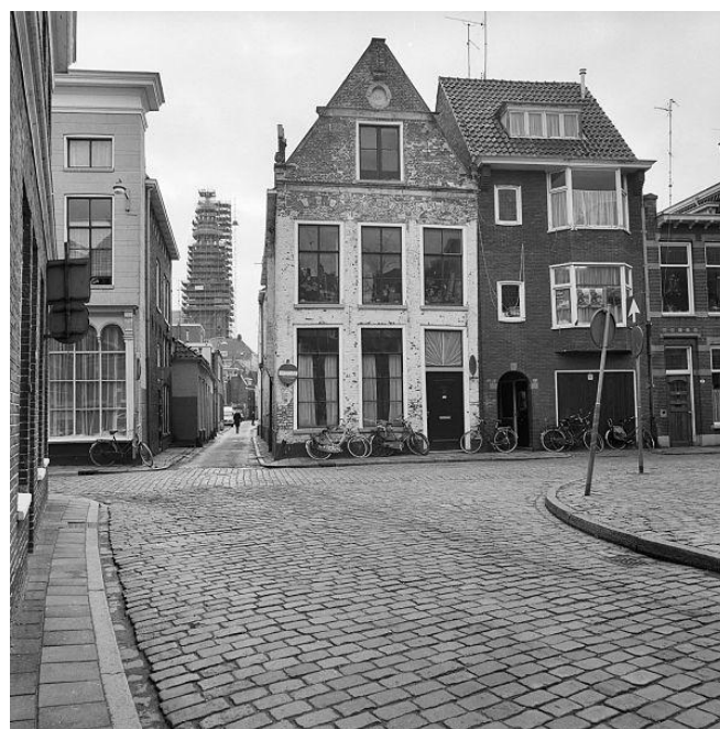
This narrow street (Lutkenieuwstraat) was aimed to become a main street https://commons.wikimedia.org/wiki/File:Overzicht_Turftorenstr.-Lutkenieuwstr._-Groningen_-_20092377_-_RCE.jpg
