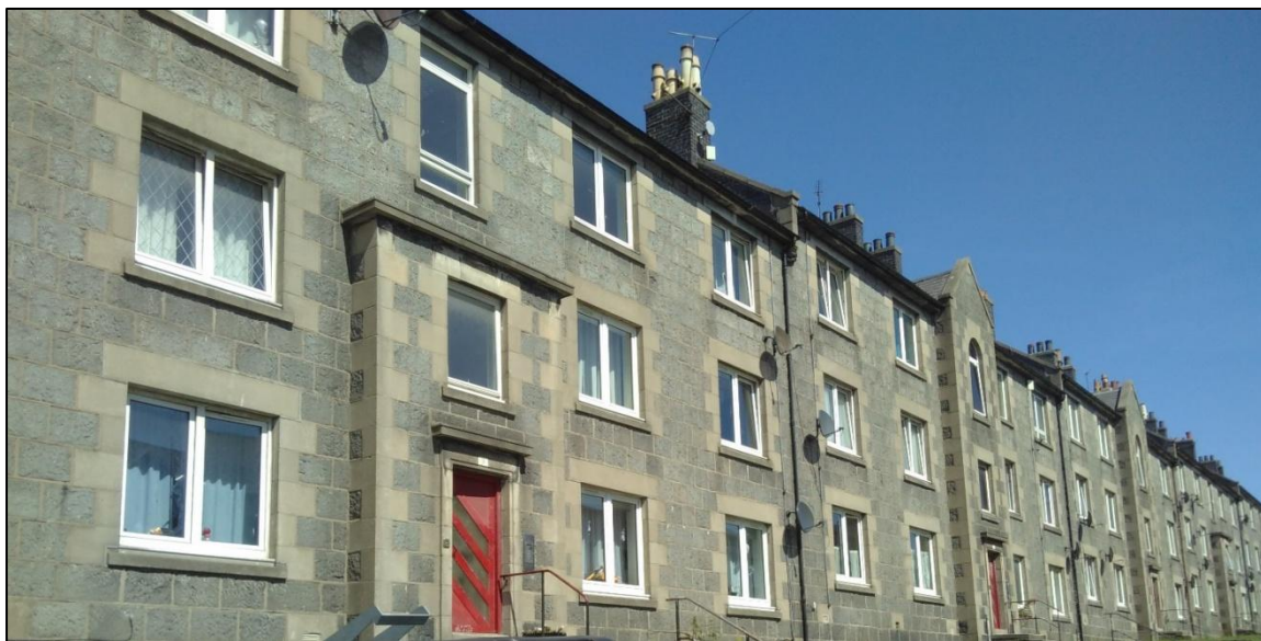
Example showing granite-built tenements in the case study area.
